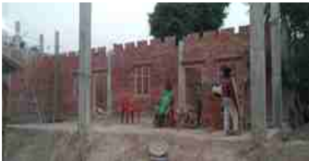
Church building under construction - Gonda
